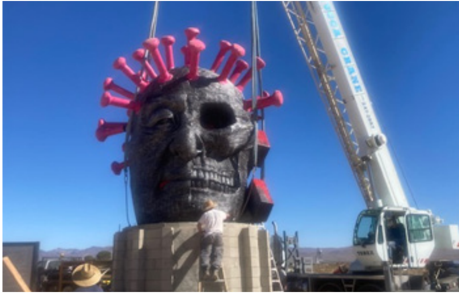
Construction crew drops Weiming Chen's replacement sculpture CCP Virus II, created less than a year after the destruction of the original CCP Virus sculpture, into place on June 1, 2022. Photo: Mark Gutglueck
