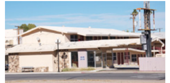
The Overland Motel today.
